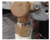
Suitable to detect pinpoint leakage. Apply bubble solution over the potential leakage point, and detect fluorocarbons blowing out from the point.
