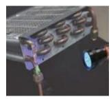
Inject fluorescent agent into tubes, and detect the leakage point by identifying the leaking agent by using ultraviolet lamp.
